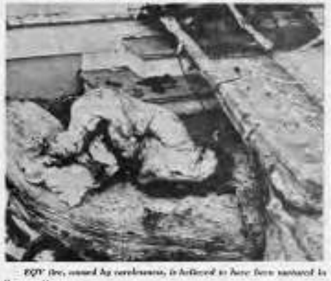
The rubble from the destroyed E.Q.V. House is shown in this photograph. The debris consists of twisted metal, broken wood, and other structural remains.
