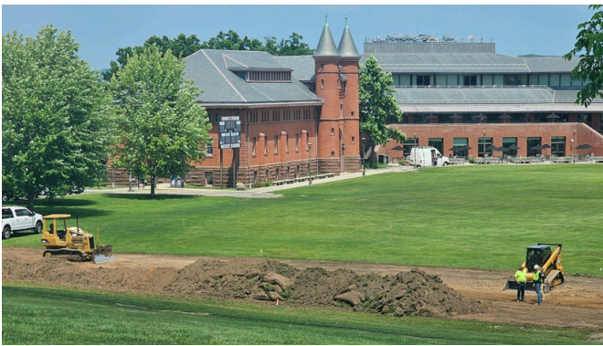
2024 installation of hot water heating pipes
